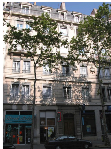
Elévation principale Phot. Maryannick Chalabi IVR82_20046904567NUCA
