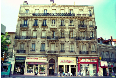
Façade principale Phot. Cendrine Sanquer IVR82_19974202089ZE
