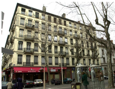
Elévation, 25 cours Suchet Phot. Chantal Archer-Galéa IVR82_20016901241NUCA
