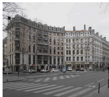
Elévation place Victor-Basch Phot. Eric Dessert IVR82_20056900636NUCA
