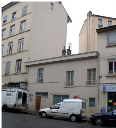
Elévation principale Phot. Maryannick Chalabi IVR82_20086900857NUCA
