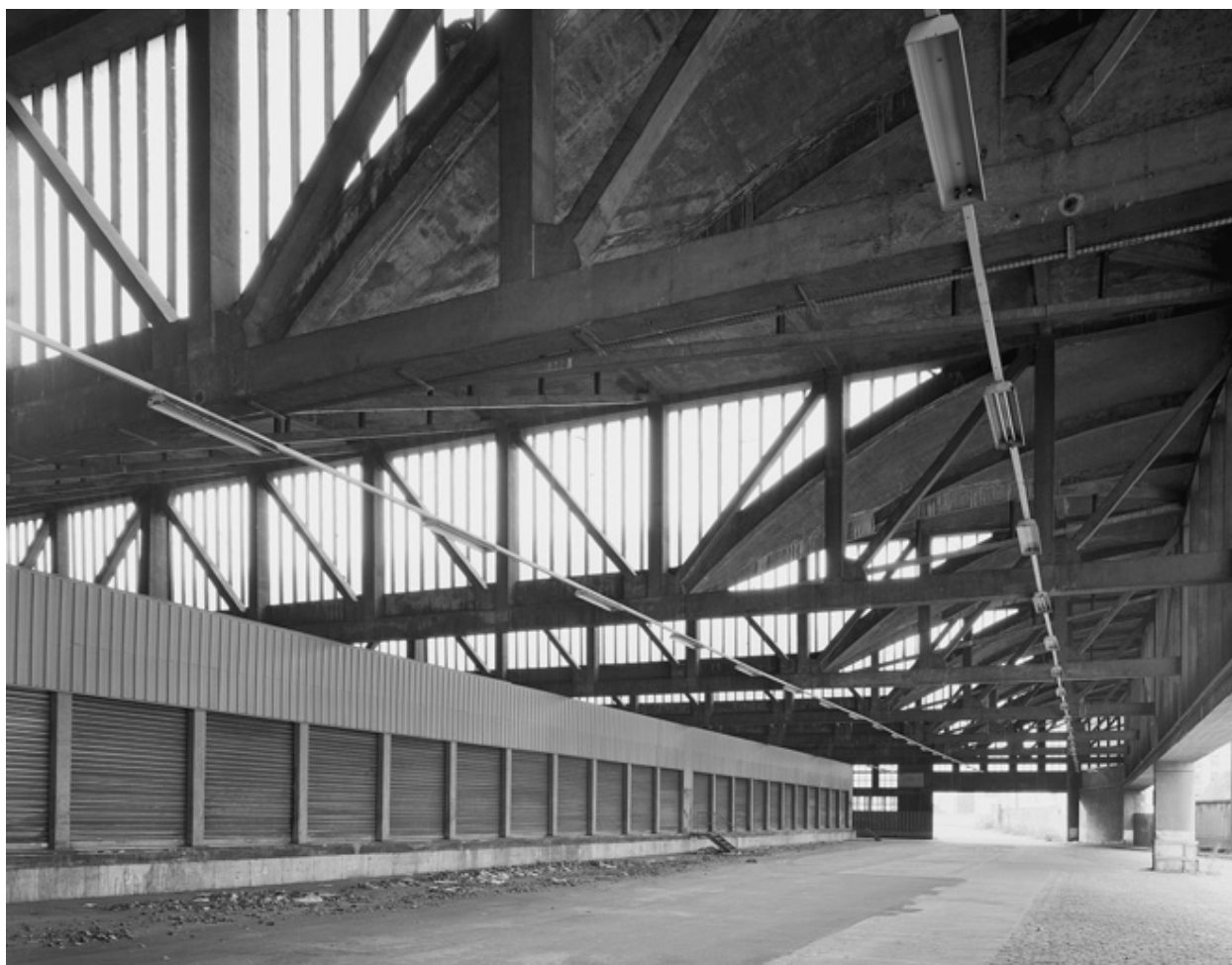
Charpente : shed structure béton
