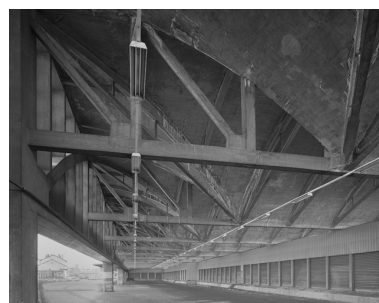
Charpente béton Phot. Didier Gourbin IVR82_20066900145V
