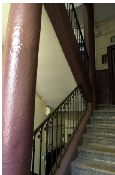
Escalier Phot. Bernard Ducouret IVR82_20036901231NUCA
