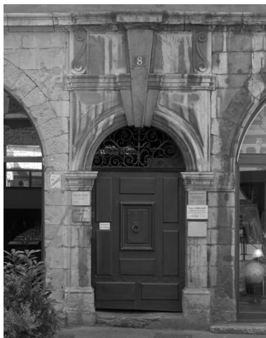
Façade, porte Phot. Didier Gourbin IVR82_20056901542NUC
