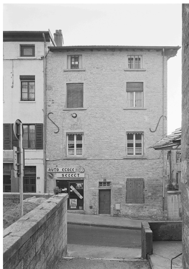
Elévation principale. Phot. Eric Dessert IVR82_19900100389P
