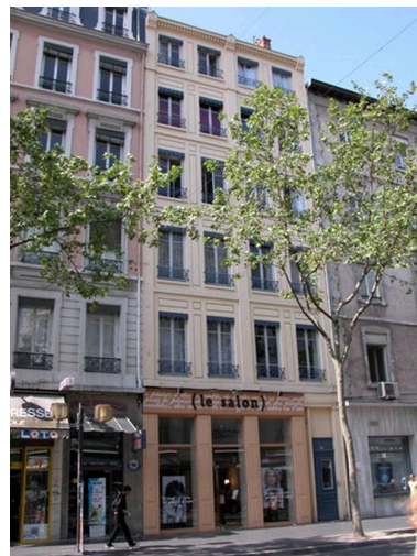
Elévation principale Phot. Maryannick Chalabi IVR82_20046904664NUCA
