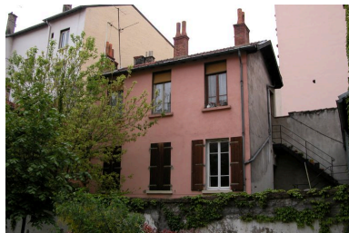
Elévation principale Phot. Maryannick Chalabi IVR82_20046904117NUCA
