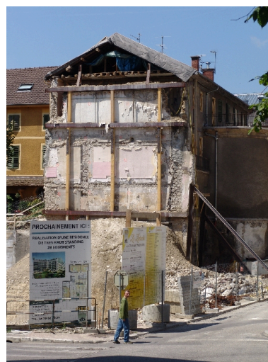
Pignon oriental Phot. François Fouger IVR82_20057300742NUCA
