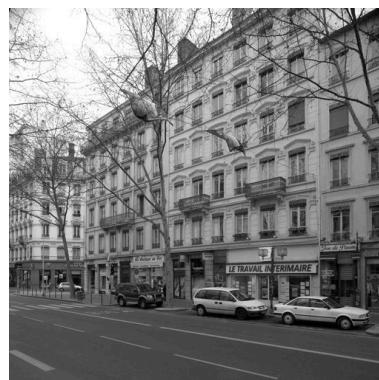
Elévation principale Phot. Eric Dessert IVR82_20056900595NUC
