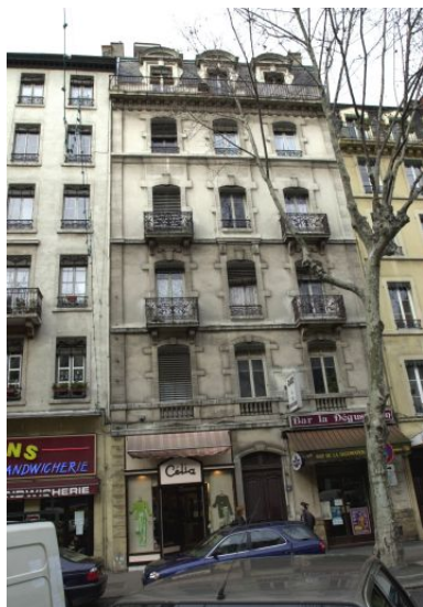
Elévation principale Phot. Maryannick Chalabi IVR82_20016900259NUCA
