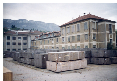
Elévation nord Repro. François Fouger IVR82_20087300696NUCB
