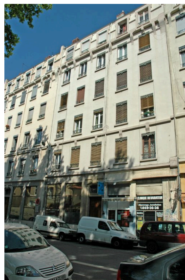
Elévation principale Phot. Maryannick Chalabi IVR82_20076900297NUCA
