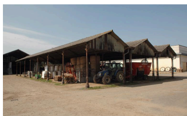
Hangar Phot. Catherine Guégan IVR82_20150100108NUCA
