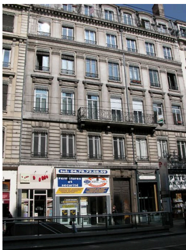
Elévation principale Phot. Maryannick Chalabi IVR82_20046904672NUCA
