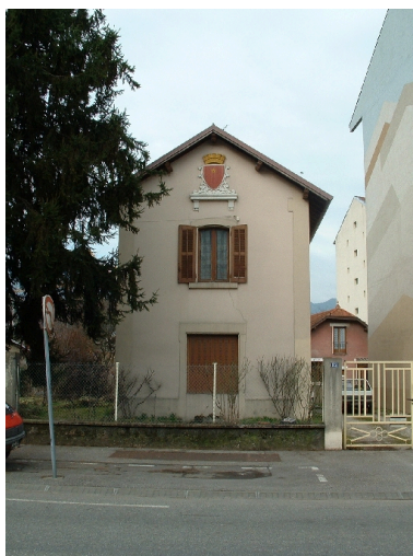
Façade-pignon Phot. François Fouger IVR82_20097300555NUCA
