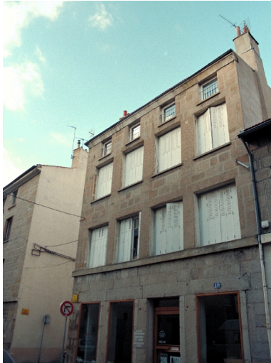
Elévation principale Phot. Cendrine Sanquer IVR82_19974201992ZE
