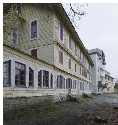
Façade principale Phot. Eric Dessert IVR82_20147302057NUCA
