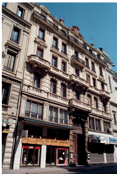
Façade principale Phot. Cendrine Sanquer IVR82_19974201836ZE
