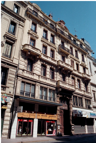
Façade principale Phot. Cendrine Sanquer IVR82_19974201836ZE
