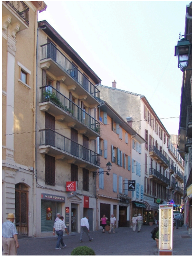
Façade Phot. François Fouger IVR82_20057300581NUCA
