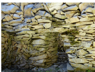
Travée est. Mur ouest. Phot. Alexei Laurent IVR84_20162601228NUCA
