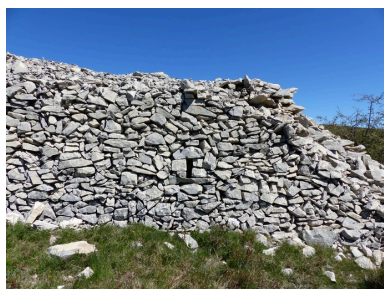
Elévation sud, partie est. Phot. Alexei Laurent IVR84_20162601218NUCA
