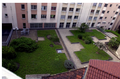
Cour-jardin, 30 rue Rachais Phot. Maryannick Chalabi IVR82_20076902061NUCA
