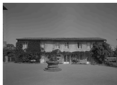
Communs, aile droite. Phot. Eric Dessert IVR82_19920100516P
