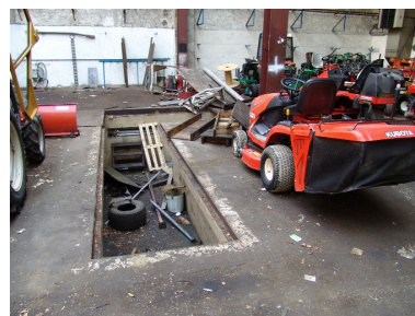
Fosse technique Phot. François Fouger IVR82_20077300509NUCA
