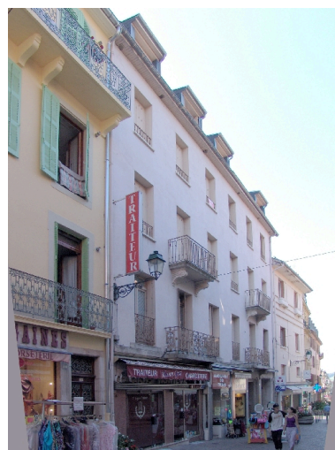
Façade Phot. François Fouger IVR82_20057300574NUCA
