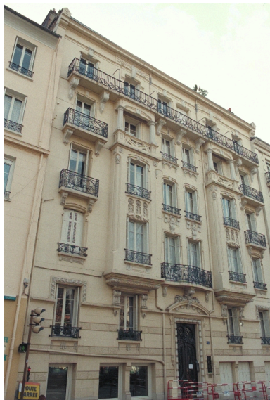
Façade principale Phot. Cendrine Sanquer IVR82_19974202018ZE
