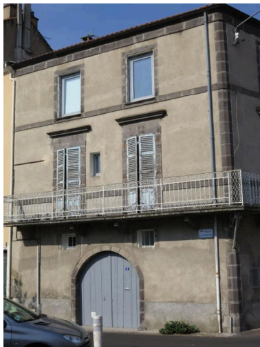
Façade principale Phot. Bruno Decrock IVR84_20206300074NUCA
