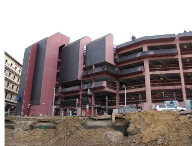
Façade Phot. François Fouger IVR82_20057300745NUCA
