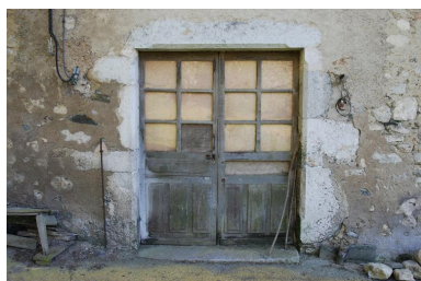
Detail of the double door on the ground floor, front facade. Phot. Thierry Monnet
