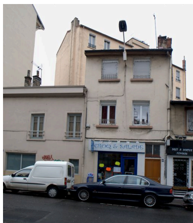
Elévation principale Phot. Maryannick Chalabi IVR82_20096901284NUCA
