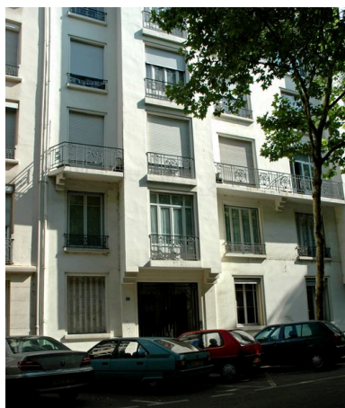
Elévation principale Phot. Maryannick Chalabi IVR82_20066903086NUCA
