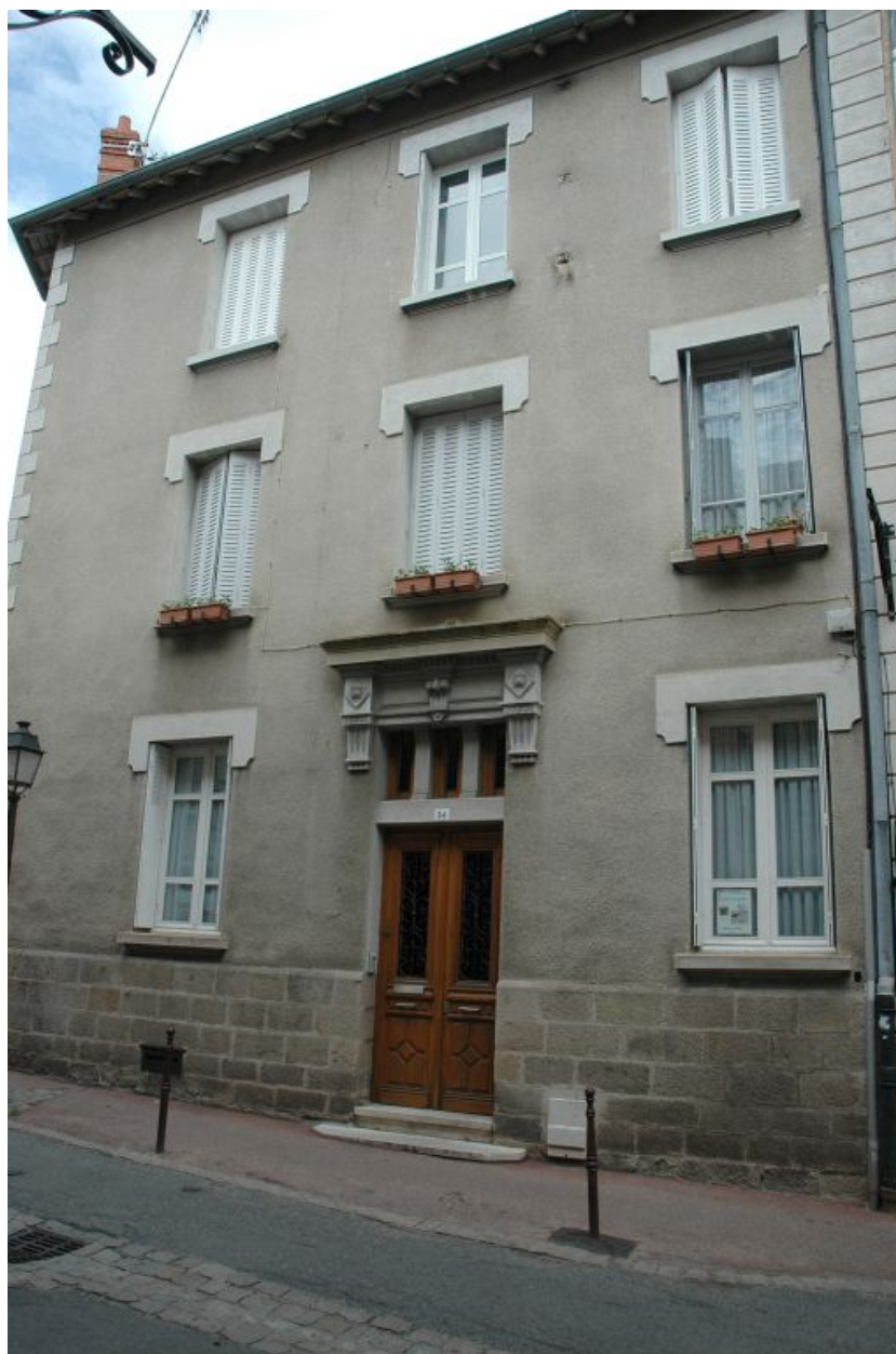
Elévation principale, rue Martin-Bernard.
