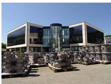
Façade principale Phot. François Fouger IVR82_20087300635NUCA
