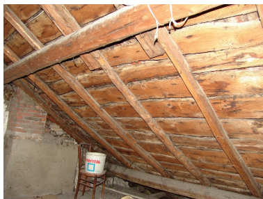
Charpente Phot. François Fouger IVR82_20047300514NUCA
