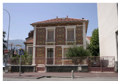
Façade Phot. François Fouger IVR82_20067300653NUCA
