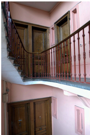
Portes palières Phot. Maryannick Chalabi IVR82_20106905113NUCA
