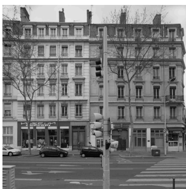
Elévation principale Phot. Eric Dessert IVR82_20056900630NUC
