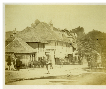
Halle aux ânes Repro. François Fouger IVR82_20087300279NUCB
