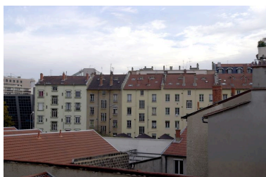
Elévation postérieure Phot. Maryannick Chalabi IVR82_20086900643NUCA
