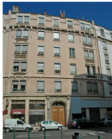
Elévation principale Phot. Maryannick Chalabi IVR82_20076900303NUCA
