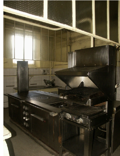
Cuisines Phot. François Fouger IVR82_20047300064NUCA
