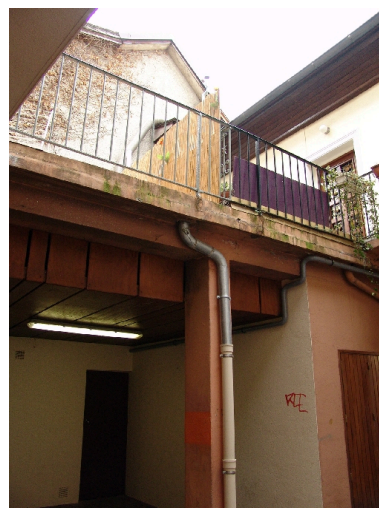
terrasse Phot. François Fouger IVR82_20047300328NUCA
