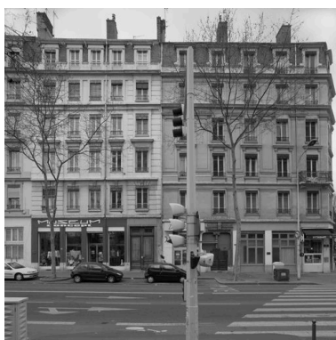
Elévation principale Phot. Eric Dessert IVR82_20056900630NUC
