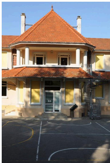
Corps central Phot. Denys Harreau IVR82_20147301266NUCA
