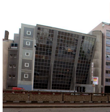
Façade principale Phot. Maryannick Chalabi IVR82_20086900763NUCA
