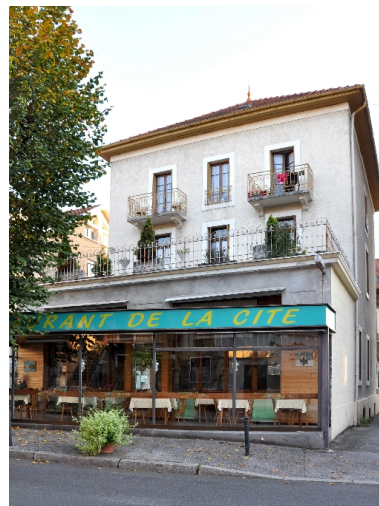
Façade Phot. François Fouger IVR82_20097301079NUCA
