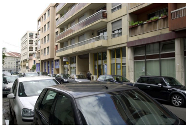
Elévation principale Phot. Maryannick Chalabi IVR82_20076902066NUCA
