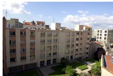
Elévation postérieure Phot. Maryannick Chalabi IVR82_20076902067NUCA
