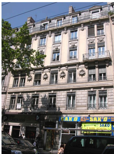
Elévation principale Phot. Maryannick Chalabi IVR82_20046904578NUCA
